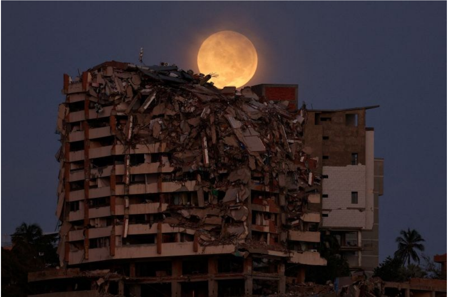
A full moon is seen behind a collapsed residential building damaged in the June 24 earthquakes, after a lunar eclipse, in La Guaira, Venezuela, August 28. REUTERS/Gaby Oraa
